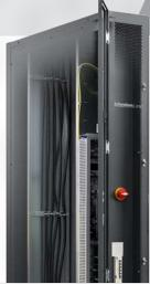
With **DataPower**, depending on the system architecture, it is possible to power the (single-phase/three-phase) PDUs, air-conditioning systems with single or redundant power supply, and monitoring systems such as presence, smoke/fire or flooding sensors; it is also possible
