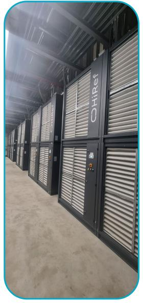
consumption. The large surface area of the finned coil heat exchanger ensures effective thermal transfer, minimizing the thermal approach between the incoming air and outgoing water, thereby maximizing overall system efficiency.
